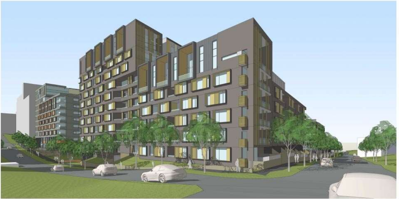
Figure 4. View from Nancarrow Avenue and Bowden Street.
